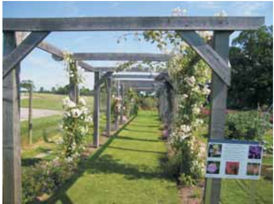
Pergola made from oak timber from Ickworth Park
